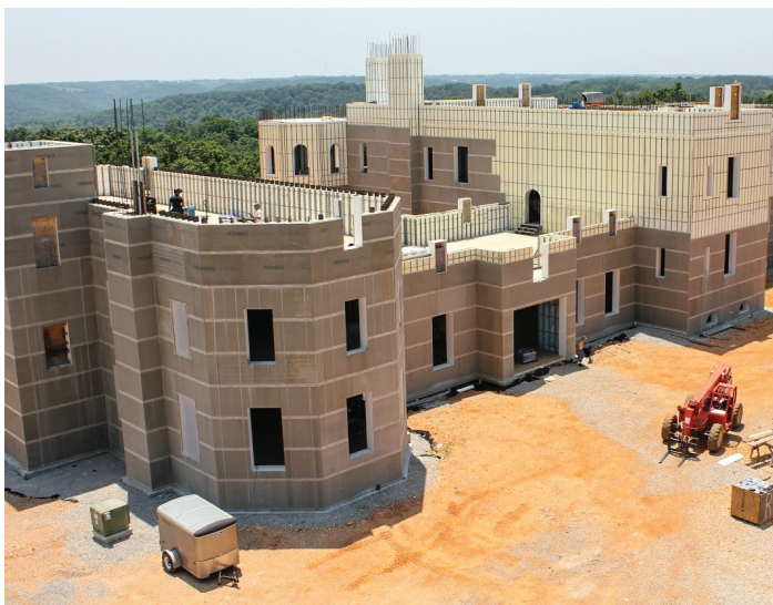
Huff is building Pensmore (above) as a showcase for his construction technology. The buildings are designed to withstand most earthquakes and F5 tornadoes.
