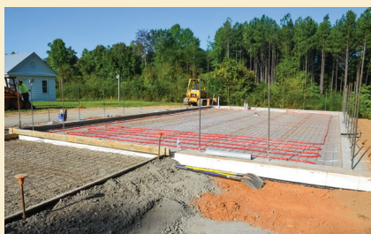
CONSTRUCTION OF THE NEW ENERGY LABORATORY
