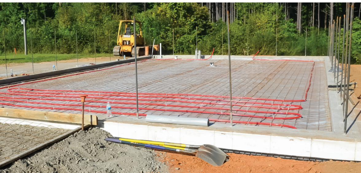
Groundwater will be pumped through tubing in the floor and walls to help maintain temperatures inside the building.
