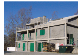
The burn building in Blackstone, where training exercises are held.
