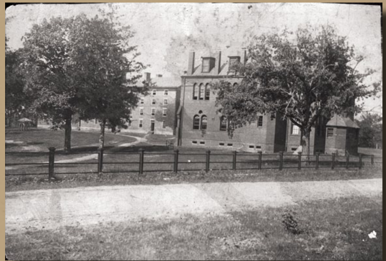
McIlwaine Hall, and behind it Cushing, as seen from the southeast from the yard in front of College Church. Note the original Cushing belfry to the far left.
