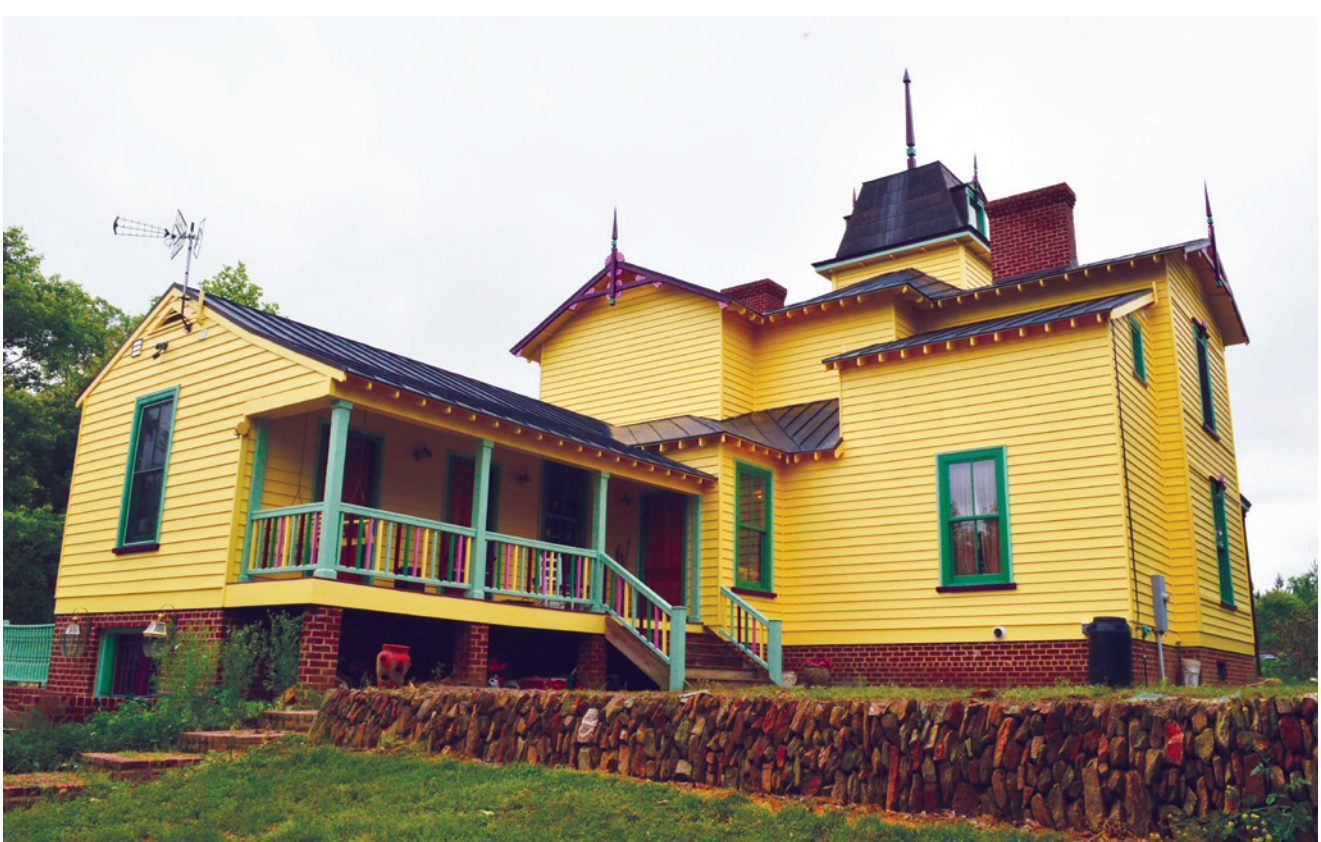
Johnson used an old-fashioned type of dry-stacked retaining wall in his backyard. The colorful house is oriented in the same direction as it was in 1875.
