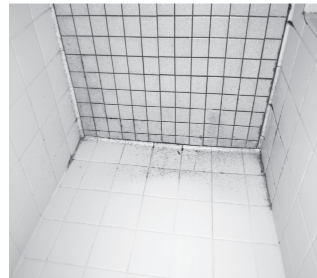
Alleged mold in a shower on Chi Phi's grounds (Photo: John David Gooden)
